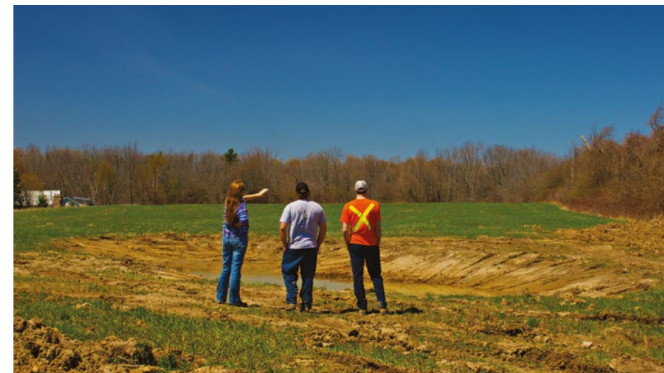
An ALUS Program Coordinator works with a landowner and a contractor during the establishment of a dug-out wetland project.
