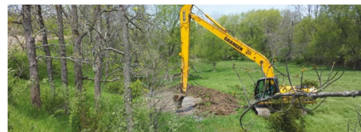
Creation of dug-out wetlands requires excavation equipment.
